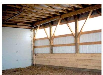
AYR-FOIL™ helps to solve or limit two of the major problems associated with post frame buildings. The reflective side of AYR-FOIL™'s prevents temperature increases providing a more comfortable environment for workers and livestock. In addition, the air bubbles reduce condensation problems. Furthermore, the white polyethylene side is easy to clean and has a bright shiny finish.
