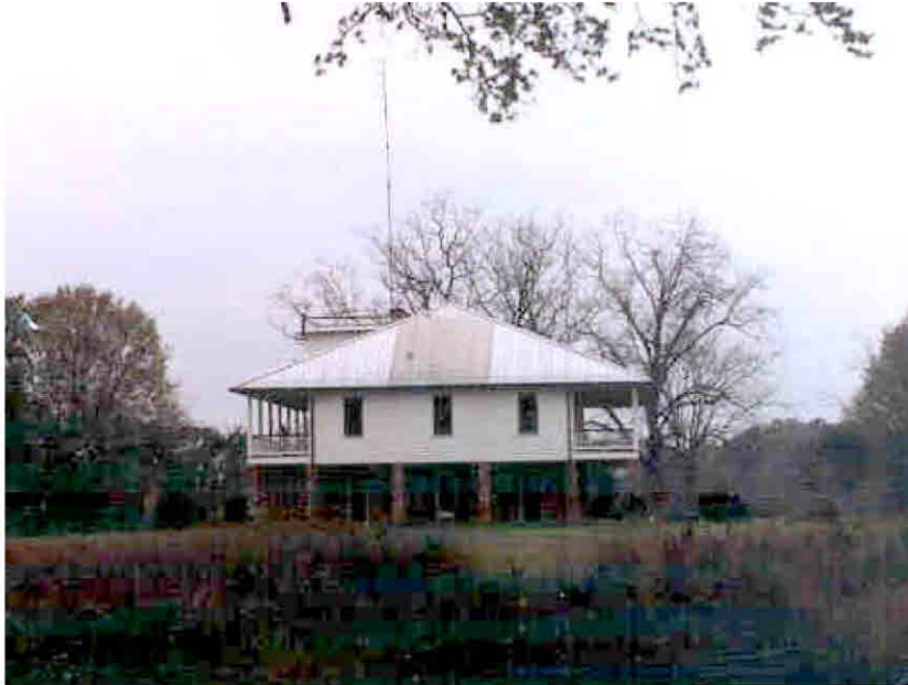
Figure 39. Differential darkening of bare GALVALUME® panels on a high slope roofing application.
