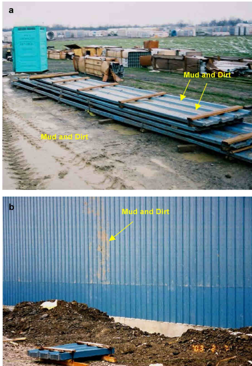
Figure 2. Photographs of mud and dirt on the prepainted GALVALUME® siding panels (a) before and (b) after the installation.
