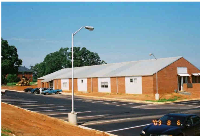
Figure 40. Differential darkening of ACRYLUME® panels on a high-slope roofing application.
